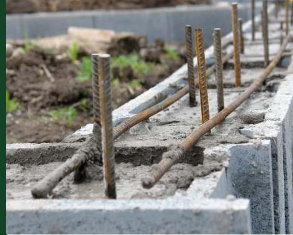
**Concrete is very strong in compression, yet very weak in tension. Steel is just the opposite – very strong in tension and very weak in compression. Because of these differences, concrete and steel form an incredible strong and durable building material when used together.**
